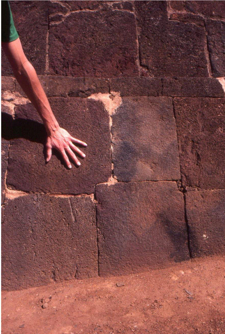
Figure 43. The facing of the major Purépecha structures at Tzintzuntzan consists of finely cut and fitted stone slabs reminiscent of the façades of temples we had earlier seen both in Bolivia at Tiahuanaco and in Peru at Cuzco and Machu Picchu. Their distinctive language and early acquaintance with metallurgy also strongly supports a possible South American origin.
